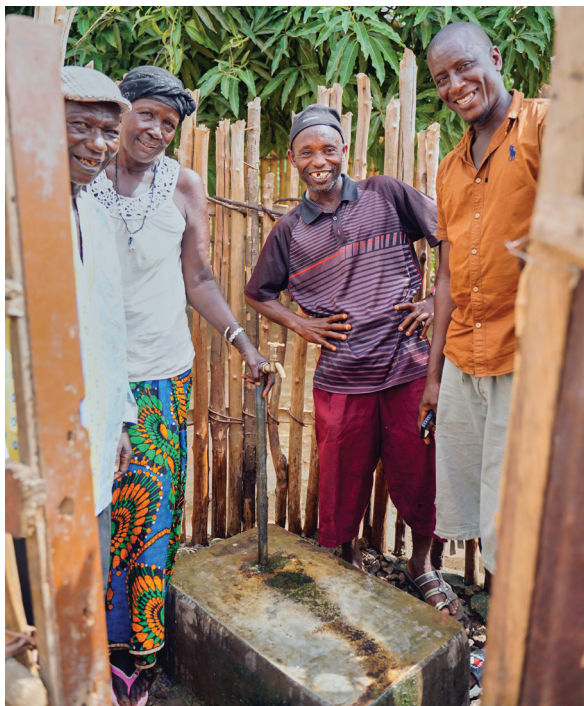
FMC and VSLA members in Mawoma repair the PHU water tap.
