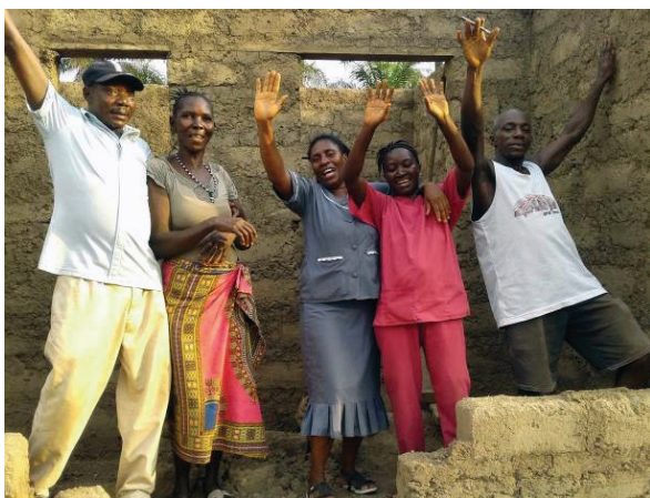
Community members constructed staff quarters at Kabonka CHP in Bombali.
