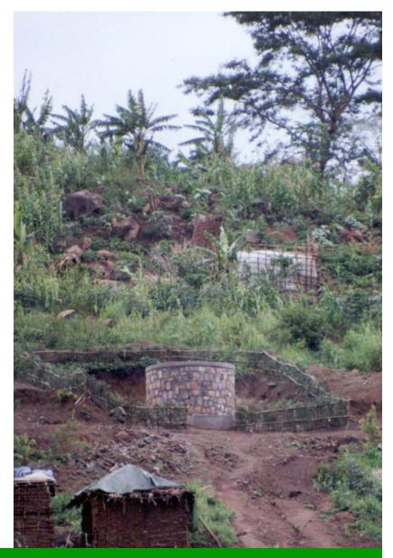
Here is a photo of the reservoir that stores water from the spring. From here the water flows down a pipe to the water points in our village.
